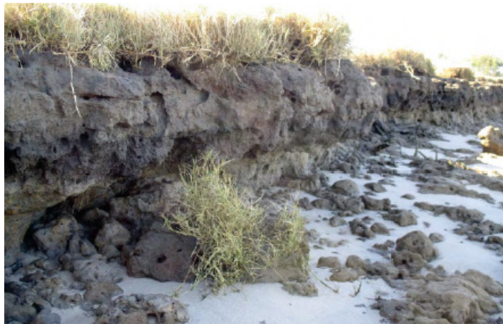
Figure 4a: Erosion at Goodwood Island
